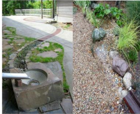
Disconnected downpipes
